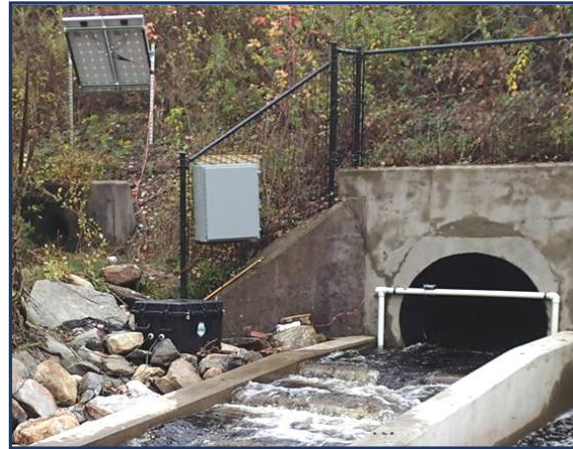
(right) Photo showing the solar power system installed adjacent to culvert outlet.
